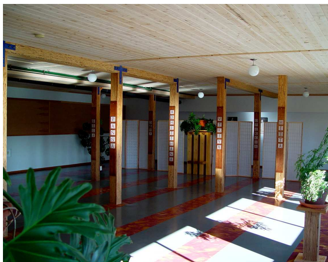
Renewed basement: pine ceiling and newly-painted walking paths.
