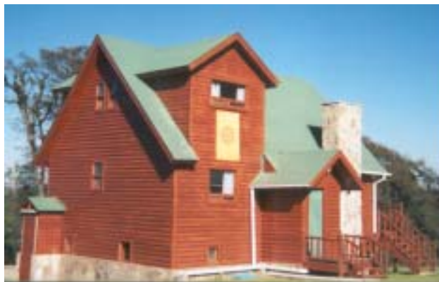
Main building, Vimutti Vihara, Mexico
