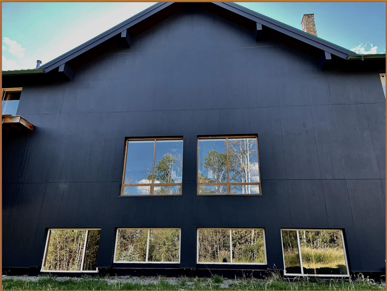
Vihara Insulation Project - East Wall
